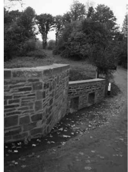
Part of the new ramparts of the bridge, with bigger side apertures to provide extra flow in extreme conditions.
